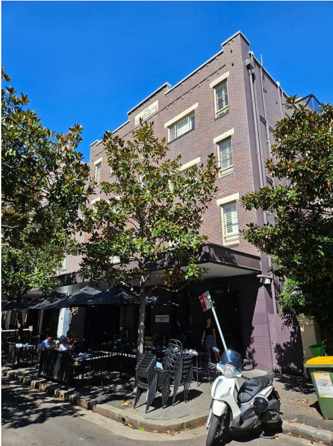
Figure 10: The 'Maisonette Hotel' building at 31 Challis Ave, viewed from the northern side of Challis Ave, facing south-east
