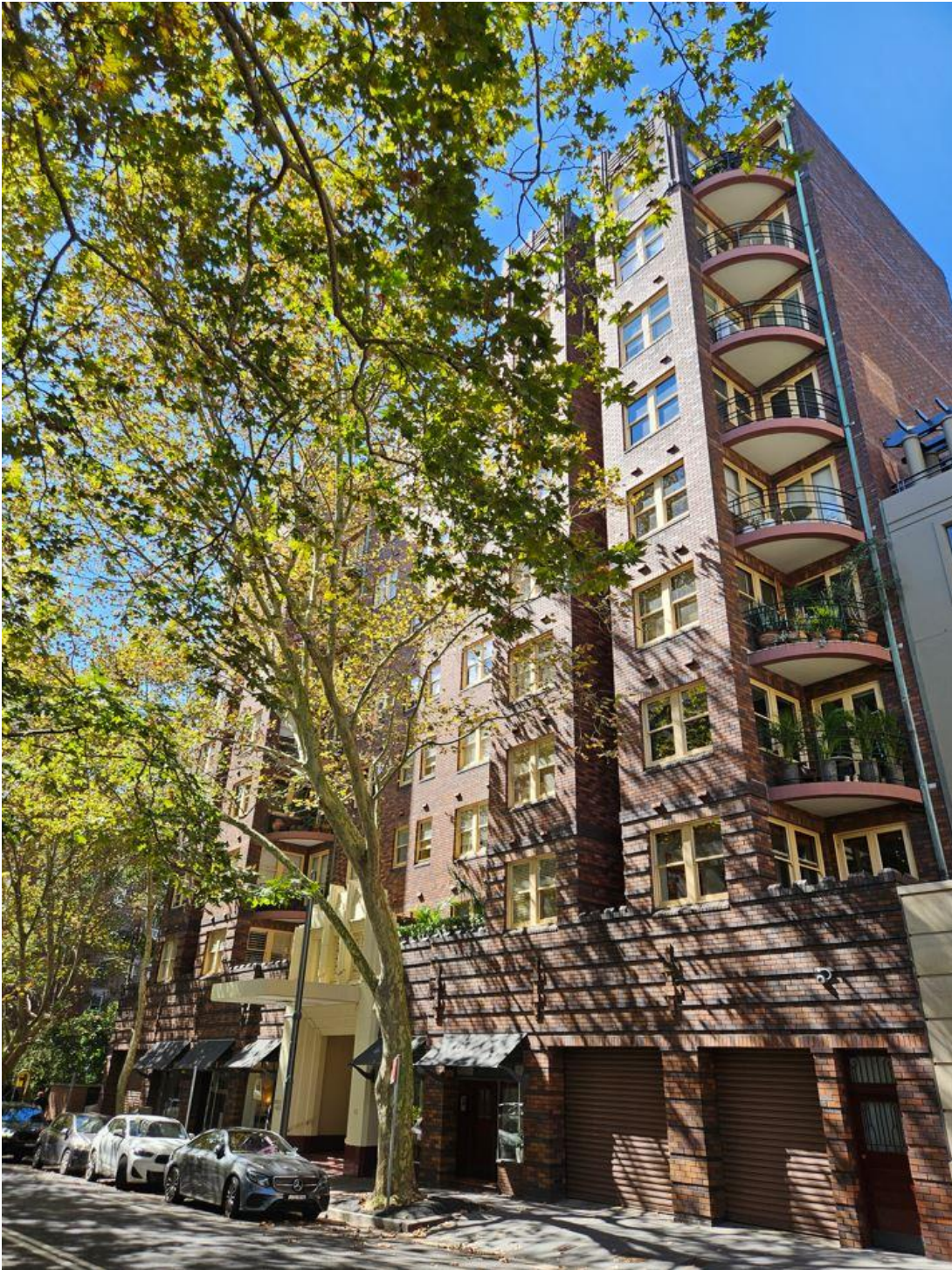
Figure 16: The 'Macleay Regis' building at 10-12 Macleay St, viewed from the western side of Macleay St, facing north-east
