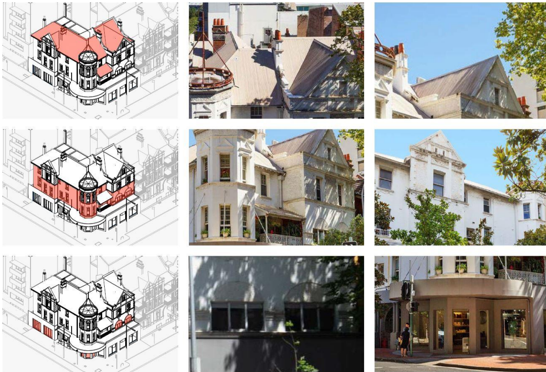
Figure 46: Three-dimensional drawing extracts and photographs of the roof (top), facade finish (middle) and non-original windows (bottom)
