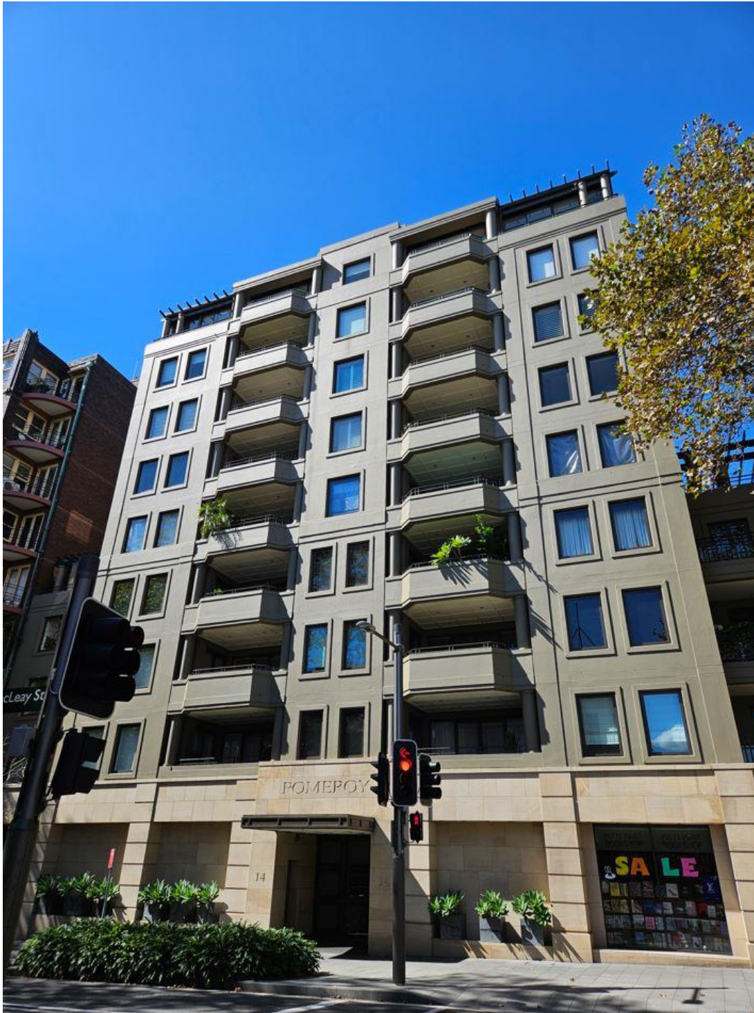
Figure 15: The 'Pomeroy' building at 14 Macleay St, viewed from the western side of Macleay St, facing east
