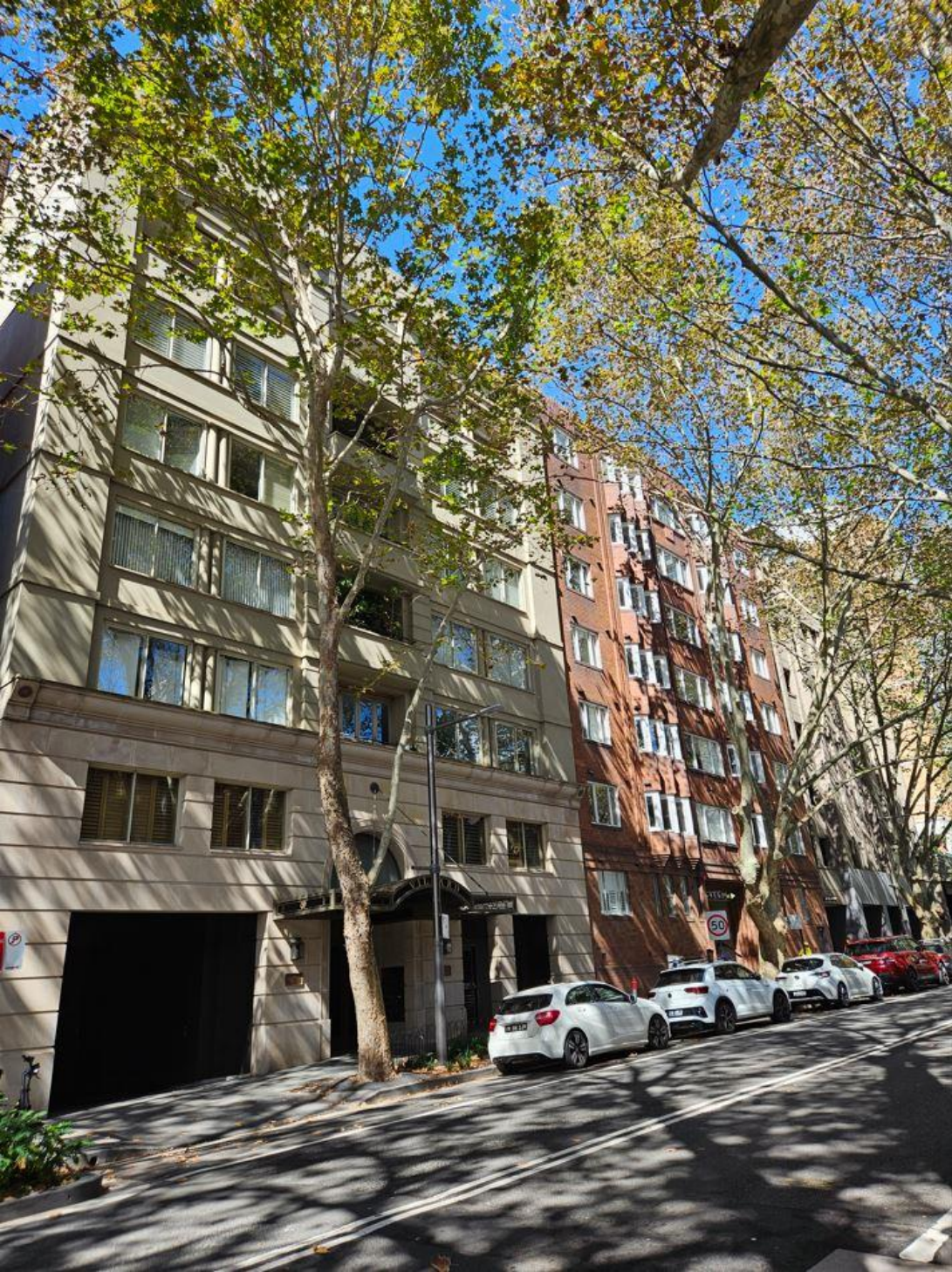
Figure 13: Existing development to the south-east of the site viewed from Macleay St, facing south-east
